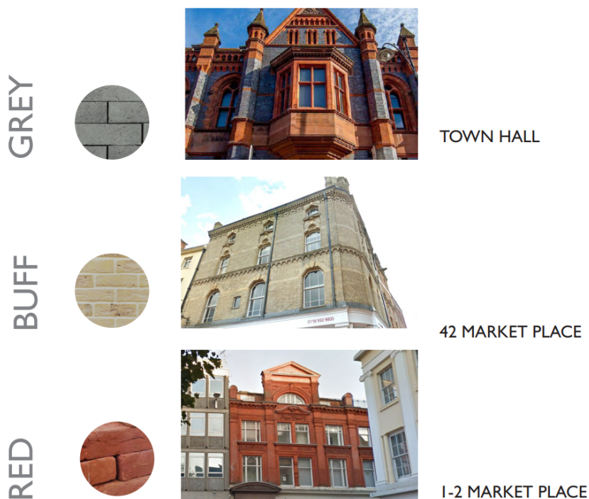
Examples of brick types found within the surrounding area
